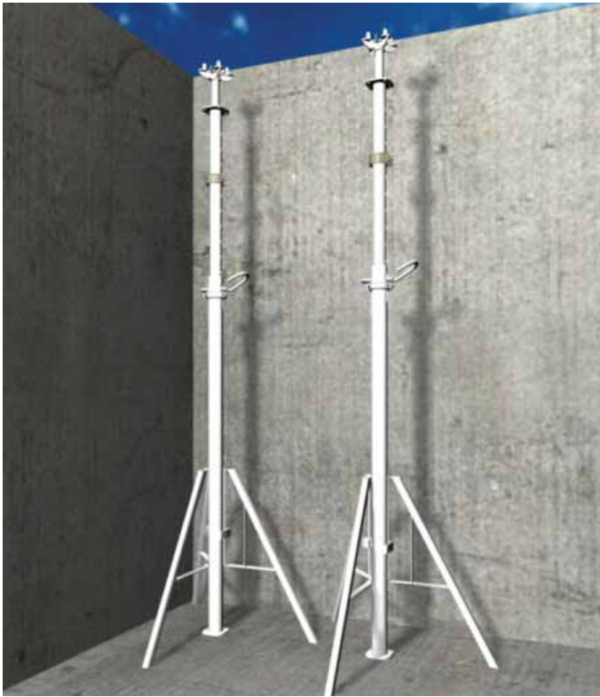
A. Position two steel props including Top Deck Bearing in the corner of the room with a distance of 90 cm and align vertically by means of Tripod Stand.
