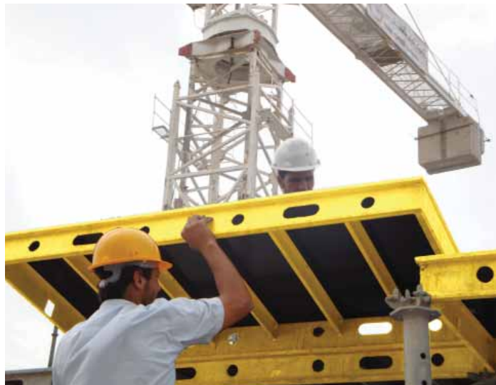
B. Support the panel in the corner using the Top Deck Bearing as illustrated.
