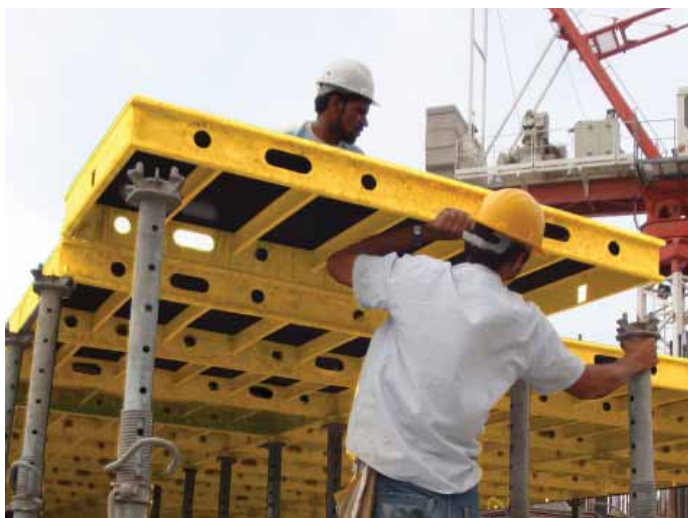
C. Final arrangement of the Alu Top Deck panels with clear positioning of the support in the corner of the panels.
